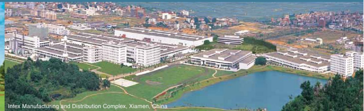
Intex Manufacturing and Distribution Complex, Xiamen, China
