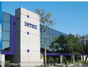
Intex Recreation Corp., Long Beach, CA, USA
