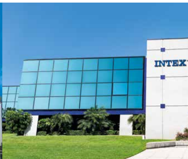
Intex Recreation Corp, Long Beach, CA, USA
