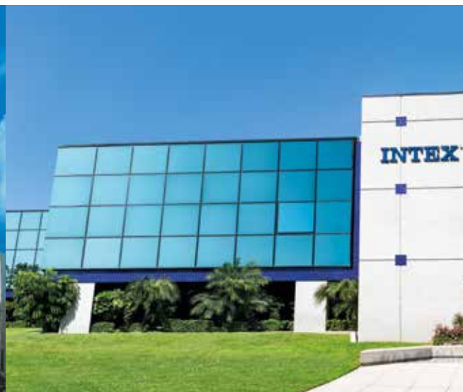
Intex Recreation Corp, Long Beach, CA, USA
