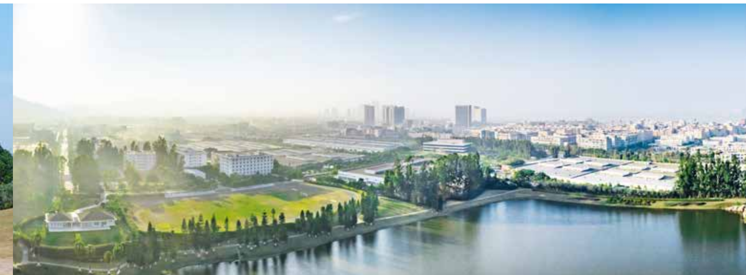
Intex Manufacturing and Distribution Complex, Xiamen, China
